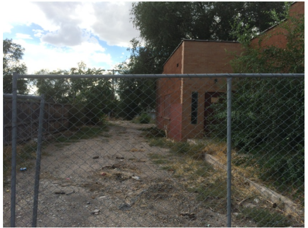
East view from 300 West
