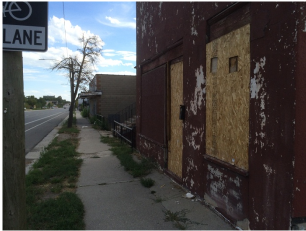
North view of sidewalk on 300 West
