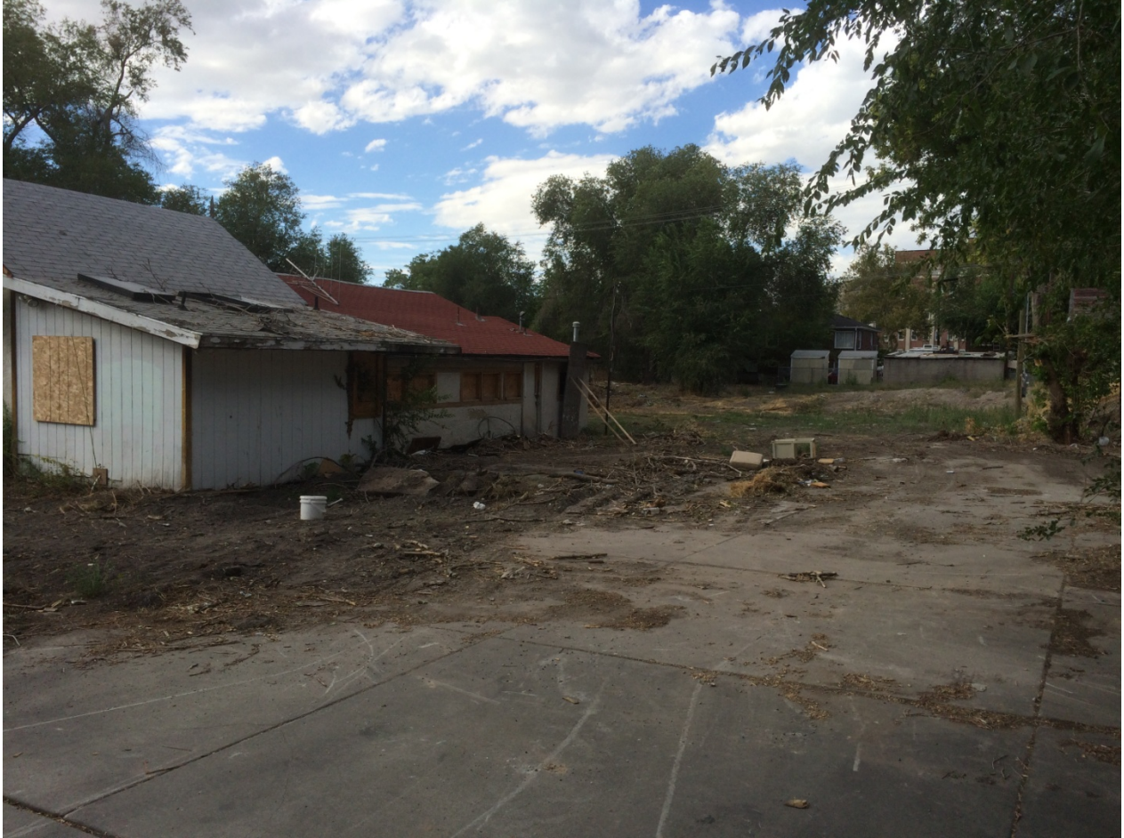
Northwest view from Reed Ave.
