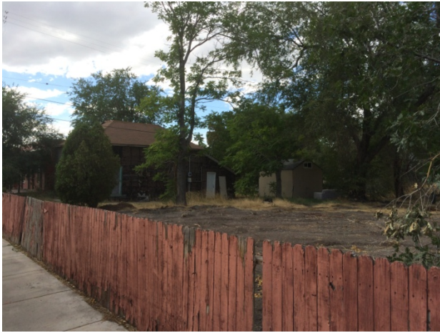
West view from Reed Ave.
